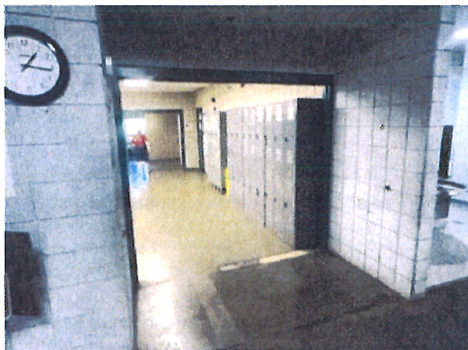
Main Locker Room -
